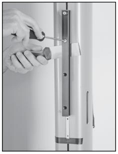
Slide slugs into place with putty knife. Loosely install 5 mm x 20 mm screws.
