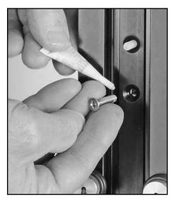
Install screw in open slug hole using blue Loctite adhesive.
