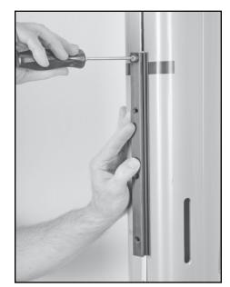
Thread 5 mm x 25 mm endstop screw through endstop, track, and into slug.
